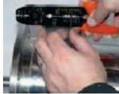
Properly remove the insulation from the motor leads and the cable leads and have a shrink hose ready with a corresponding diameter and length.
